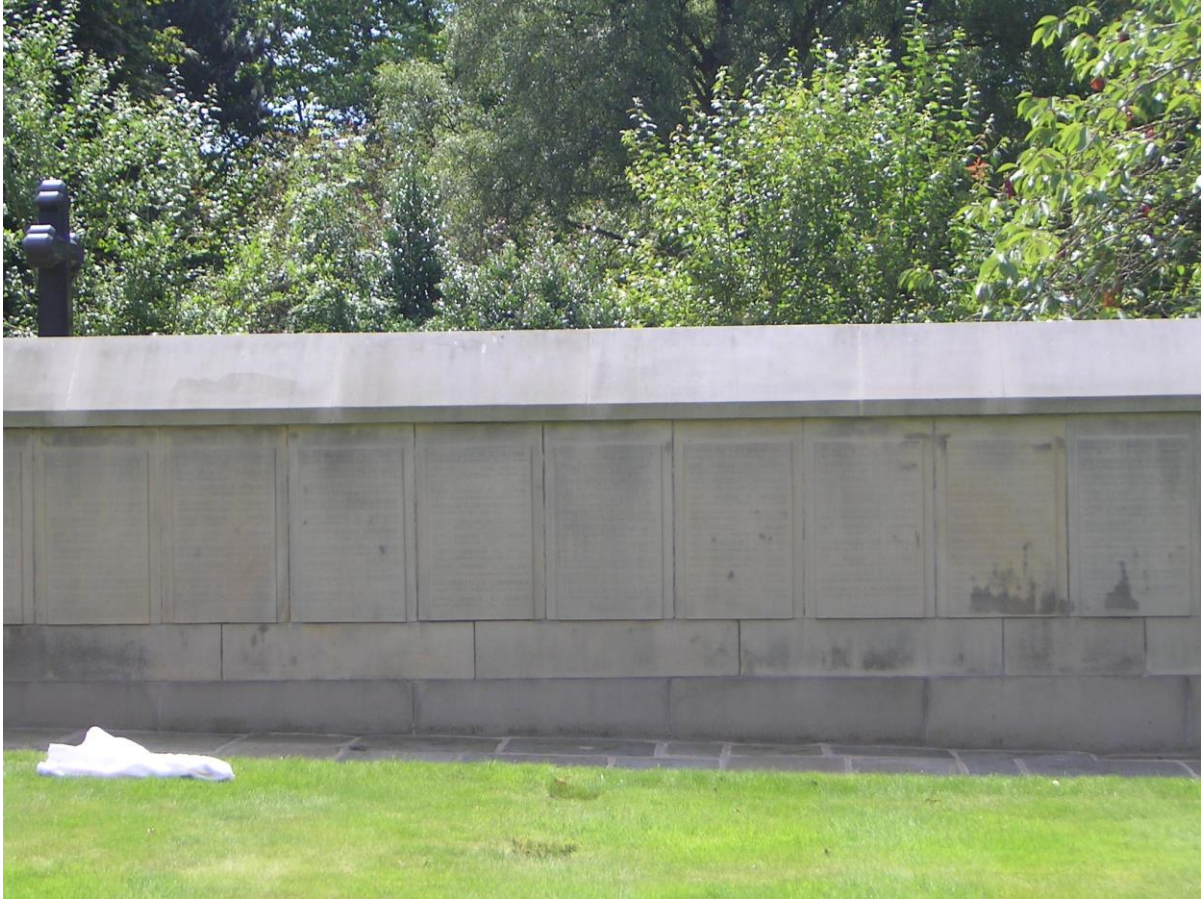
WW1 Screen Wall in Garden of Remembrance (Photo by Myra Mason – Find a Grave)
